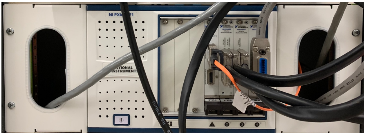
Figure 3.4.1: The PXI system (or the DAQ panel) of the UVA-NMR system
