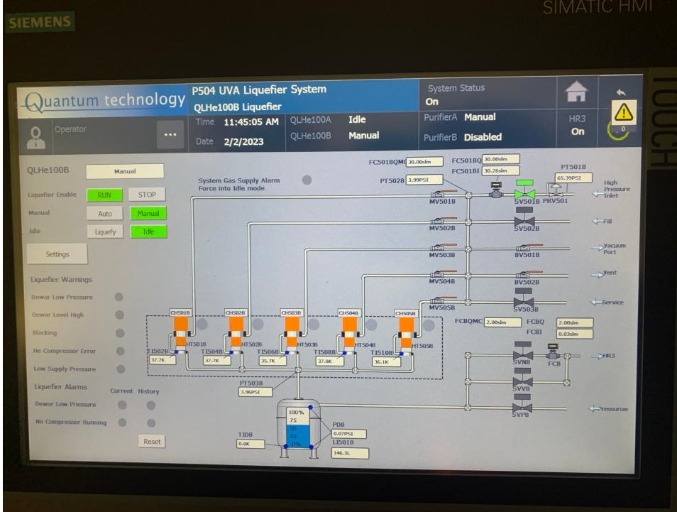
7. Set the flow on FC501(A/B)QMC to 60slm and monitor the Dewar pressure on PT503 A/B and set the flow down to 35slm and keep adjusting it until Dewar pressure is close to 5psi, and leave it with that flow.
